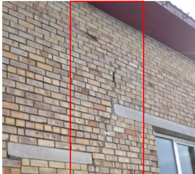
Fig. 5. Ceramic brick wall building without movement joints (photo by J.Gruntmanis)
