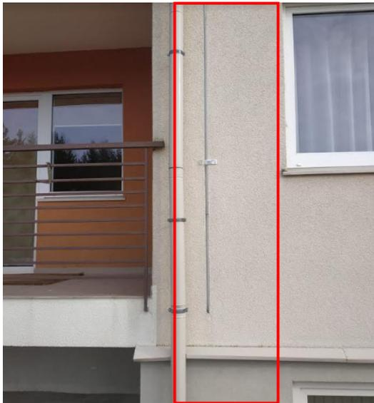
Fig. 4. Aeoroc wall block building with movement joints (photo by J.Gruntmanis)
